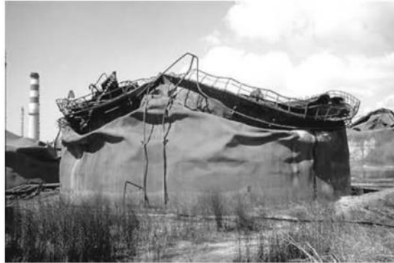
Fire damage to naphtha tanks at Tüpräs refinery.
