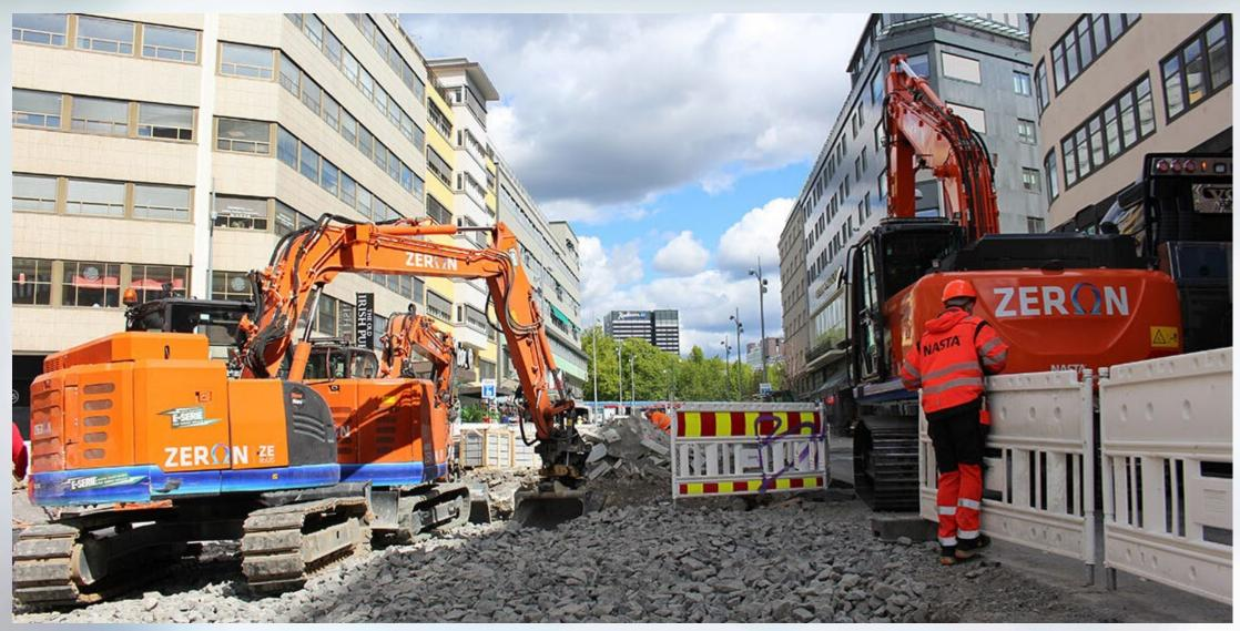
The Olav Vs Gate construction site in Oslo, Norway, is a zero-emissions project with ZERON ZE85US (9t) and ZE160LC (17.5t) electrified excavators built by NASTAAS. Courtesy of NASTAAS
