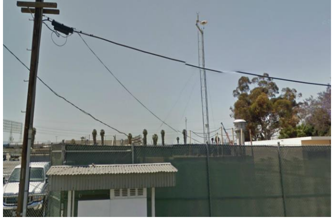
Looking at the probe from the East.
