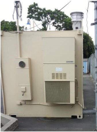
Looking at the probe from the South.
