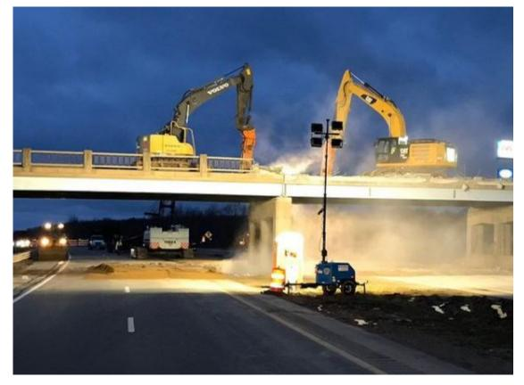
Figure 1-4 Bridge Demolition Activity Over a Large Roadway
