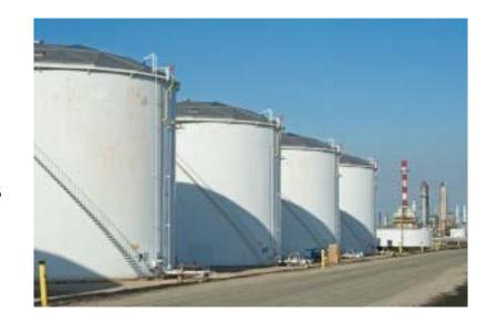
If the true vapor pressure equal to or greater than 3 psia after 2008, only current option is to dome tank
