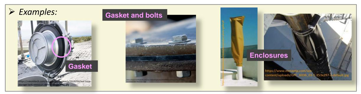
Roof opening gaps cannot exceed "visible gap" allowance of 1/8" (0.125") or must remain in vapor tight condition (<500 ppm) at all times</li>
