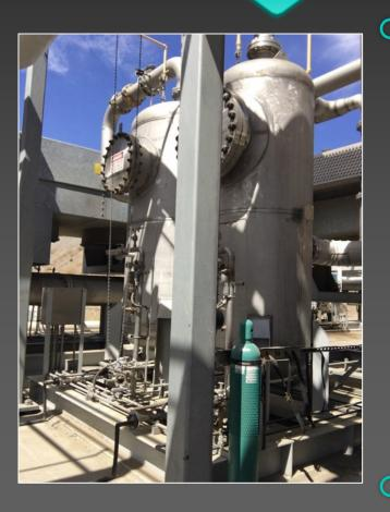
Commonly used with activated carbon as media and stored in a series of parallel canisters
