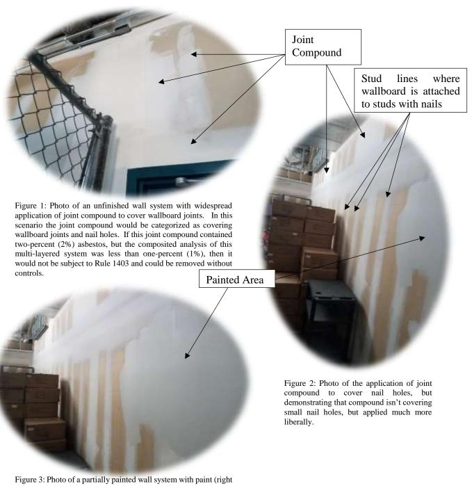
Figure 3: Photo of a partially painted wall system with paint (right side) covering joint compound and concealing where it was applied to the wall system
