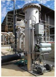
Figure 6. Nrgtek 100-SCFM Siloxane Removal System
